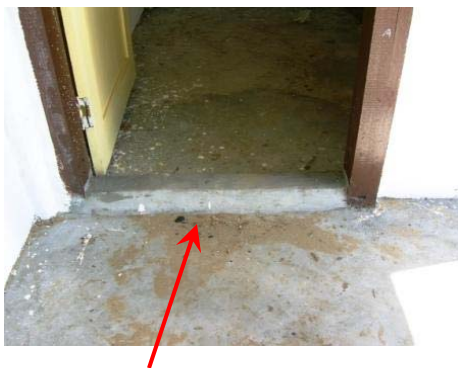
Concrete pad to the bathroom is missing
