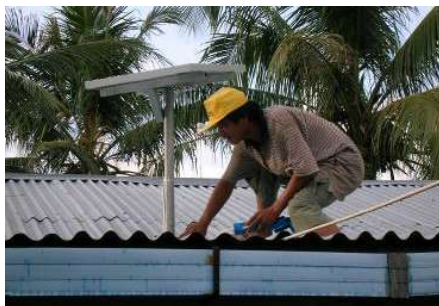
Solar panels being installed in Monaco Complex
