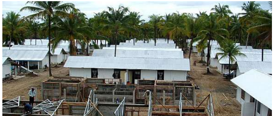
More houses under construction in the Monaco Complex
