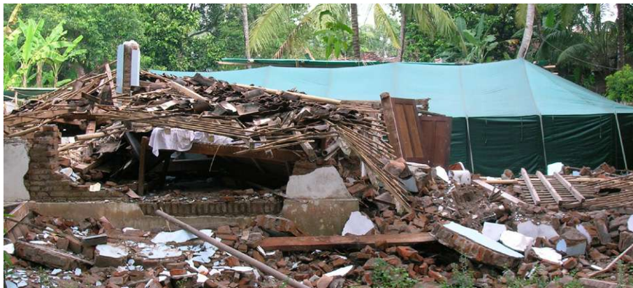
One of many homes destroyed by the earthquake in Yogyakarta
