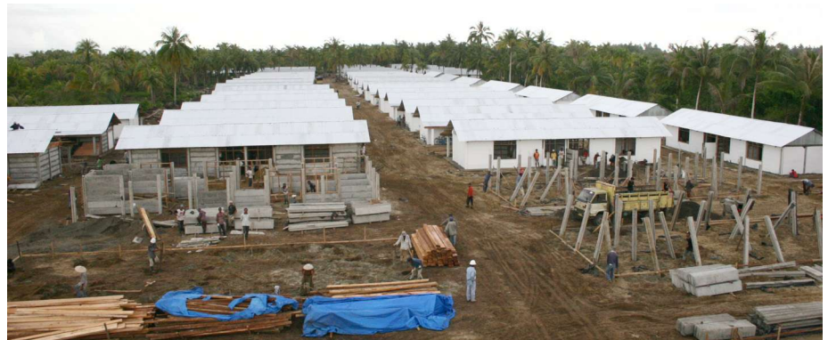
Completing the Monaco Complex in Sirombu village, Nias
